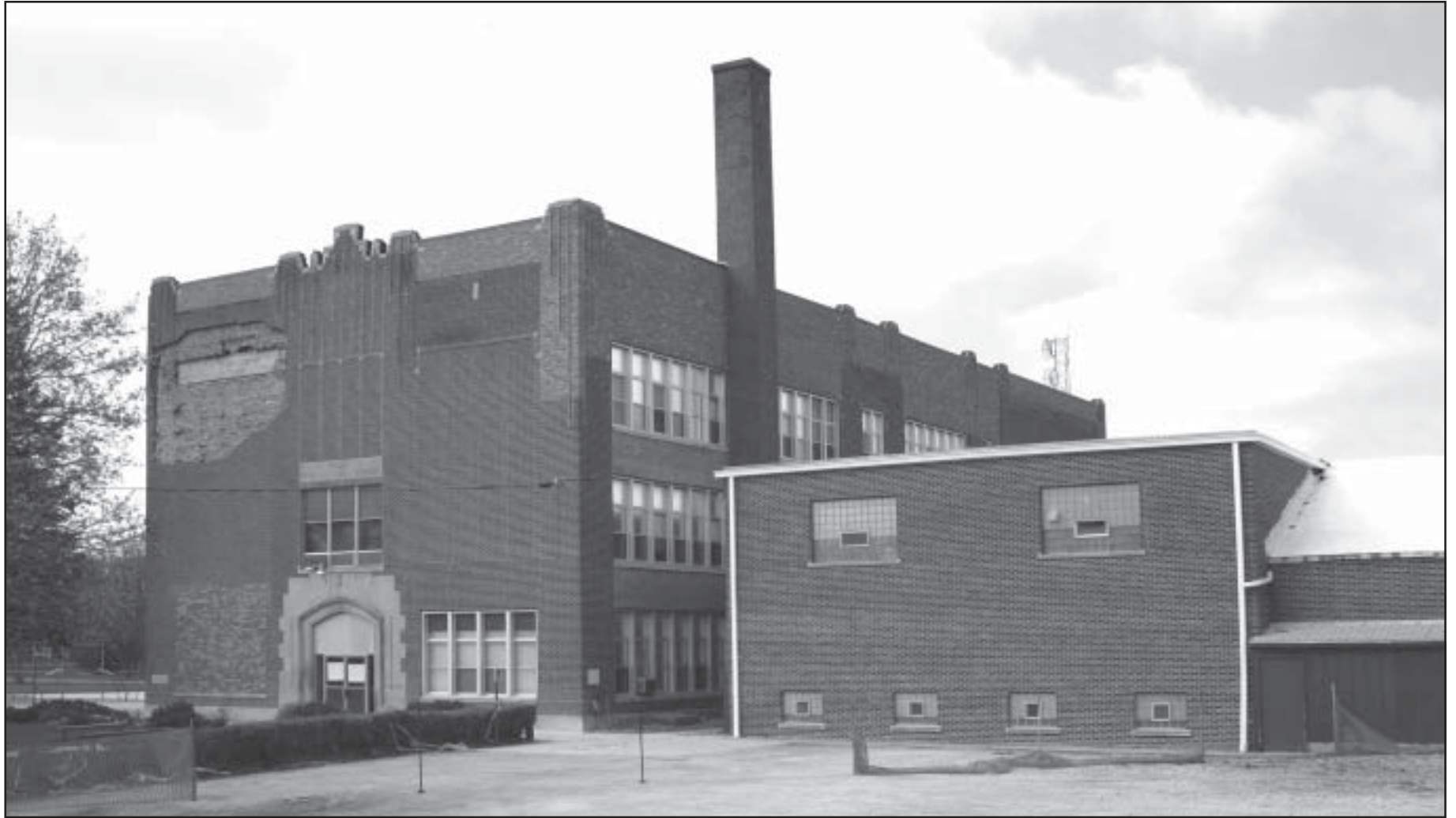
Abandoned Rolfe school building, April 19, 2004. The building on the left was built in 1907 and is scheduled to be razed.
